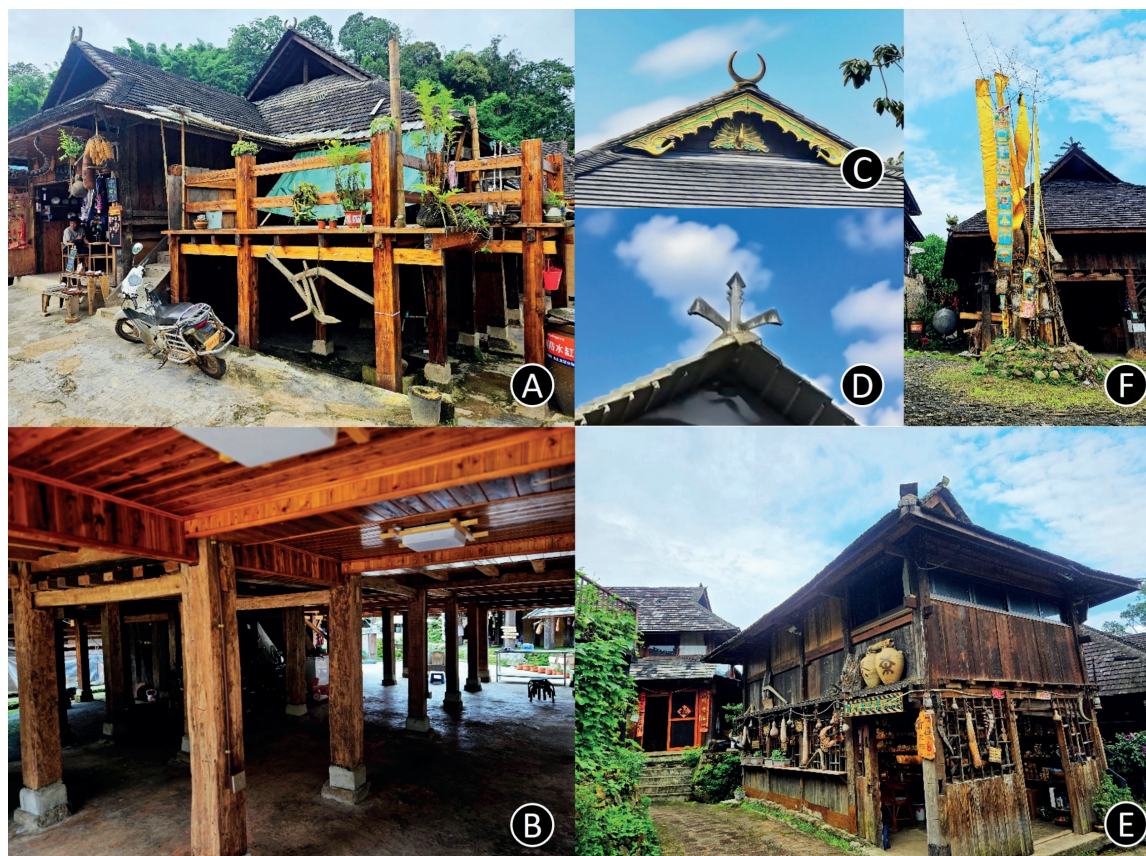
Figure 2 – Typical bamboo and timber structures in Jingmai Mountain. Traditional stilt houses of the Dai and Bulang ethnic groups, respectively (A and E). The primary building materials are wood and bamboo, with commonly used timber species including Schima spp., Quercus spp. and Pinus spp. The roofs of Dai houses typically feature double eaves and are adorned with decorative yellow ox horns at both ends of the ridge (C), while Bulang houses usually have single-eave roofs with ridge-end ornaments in the form of ‘one bud and two leaves’ (D). The lower level of the houses serves as the stilt space (B), traditionally used for storage or keeping livestock, though its function has often changed in modern times. F is the village centre, where various traditional rituals and ceremonies are held. © all pictures Chunping Xie
